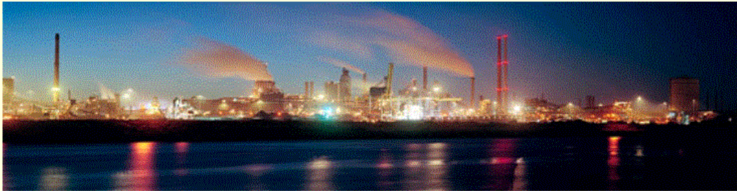
Cooling towers, chimneys
