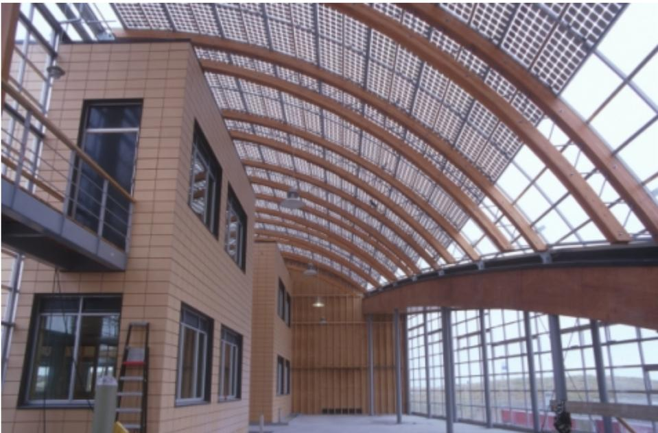
*Added value of PV: system at a newly built sustainable office building (ECN, Petten, The Netherlands, 2001. Photo courtesy BEAR Architects). PV modules fulfil multiple functions: electricity generation, roofing and partial shading.*
