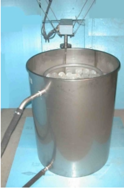
Figure 1.1 Heat storage test tank filled with PCM nodules
