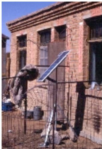
Fig 1. PV-module of a solar home system with data logger (No.3) in Sahantala, Inner Mongolia. Note the portable structure which allows transporting the module.
