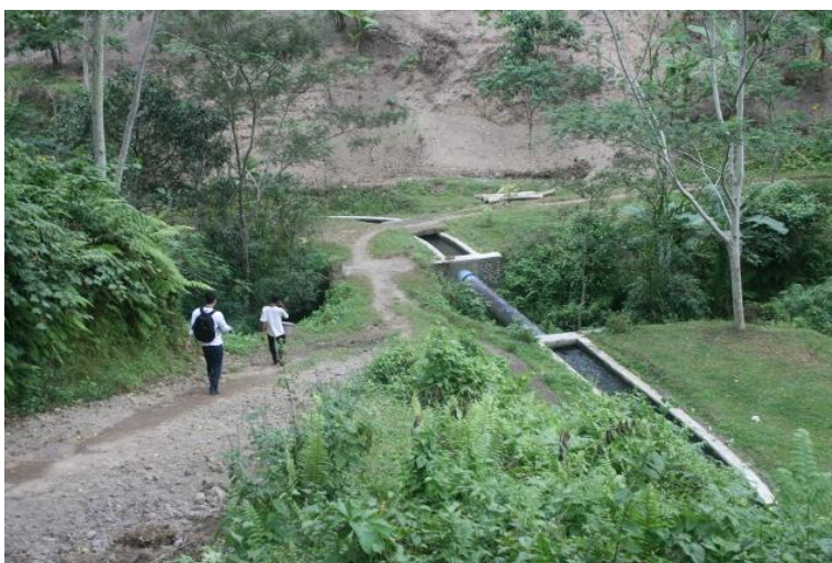
Lebah Suren micro hydropower plant, Lombok
