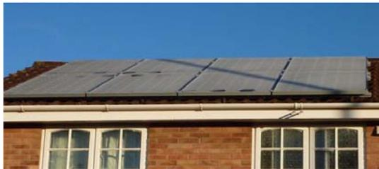
**Figure 1:** Residential PV system shaded by a lighting mast
