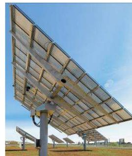
**Figure 7:** Concentrix Solar Flatcon CX-75 CPV system
