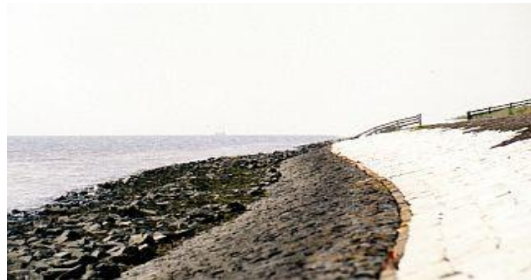
Basalt blocks used to protect sea walls
