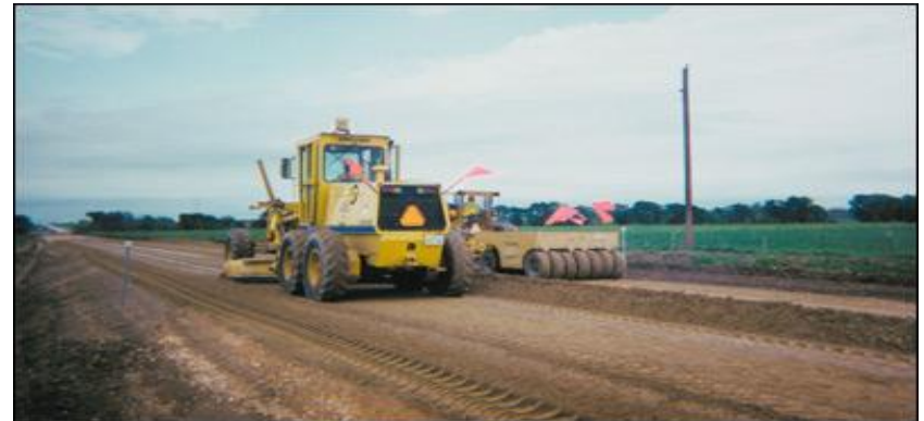
Bottom ash used in road construction
