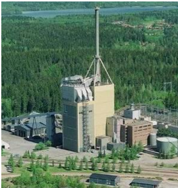
CFB FW, Lahti (Fin), co-firing PF boiler, 45 MW th_biomass
