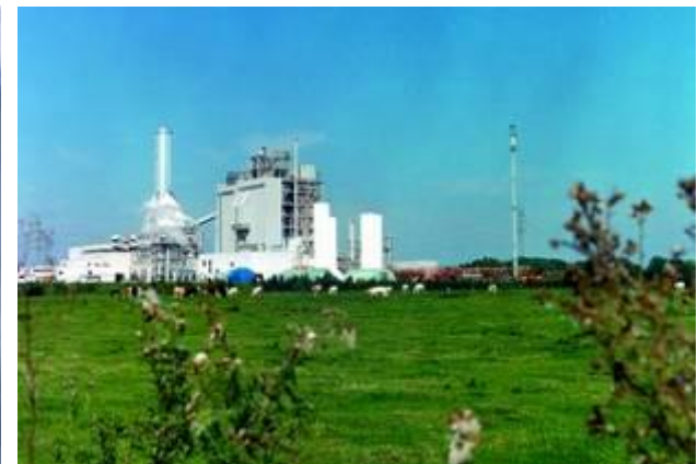
250 MW e EF gasifier up to 30wt% wood, Buggenum (NL)
