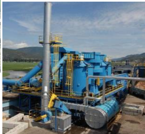
Updraft Nexterra, Tolko (Can), boiler 12 MW th_biomass
