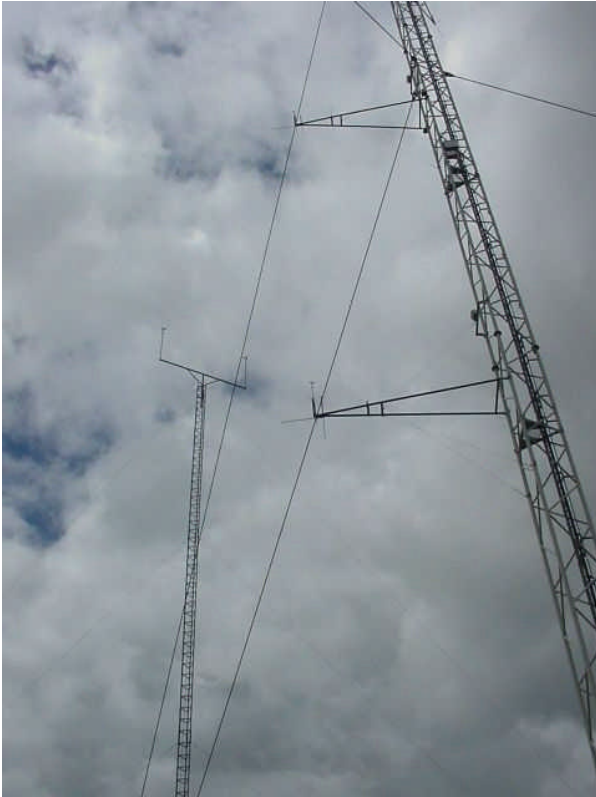
Figure 6-1. A small 25m high mast was installed next to the 108m high meteorological mast 1 at EWTW in order to assess the influence of the mast on the wind speed measurements.
