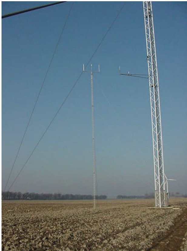
Figure 6-3. A 25m high mast was installed next to the 108m high meteorological mast 1 at EWTW. The objective of the experiment is to determine the flow disturbance of the mast on the wind speed measurements and to characterise the 2D sonic anemometer.
