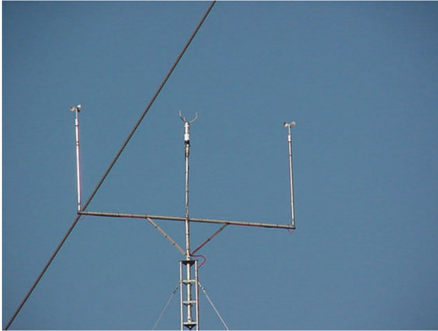
Figure 6-4. Side view of mounting of sensors on 25m mast.
