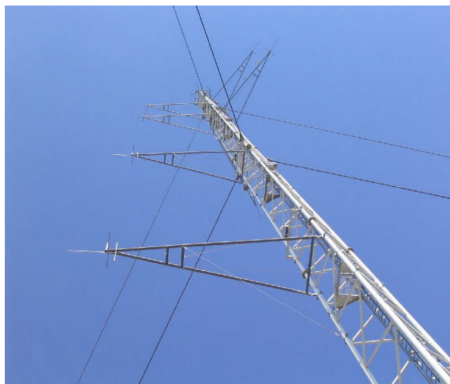
Figure 3-1 View of the meteorological mast 1 with attached booms at different levels. The booms at the lowest levels are positioned at 25m and 45m heights and are directed to East-South-East.
