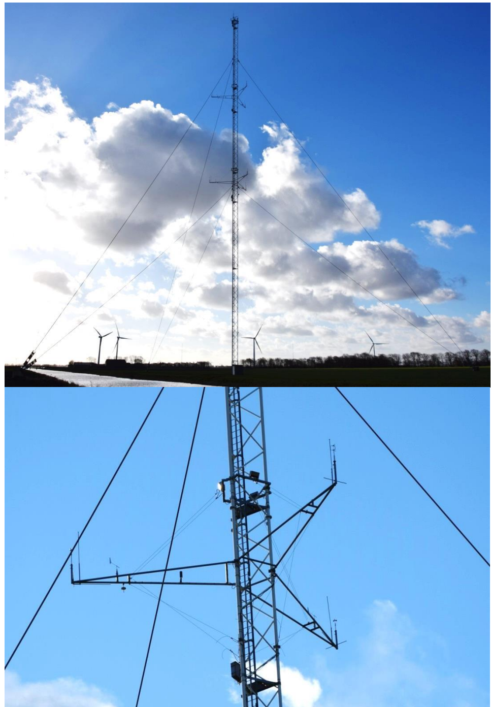
Figure 11: Lattice structure of the MM3 with attached booms positioned by guy wires [taken Jan. 2015]
