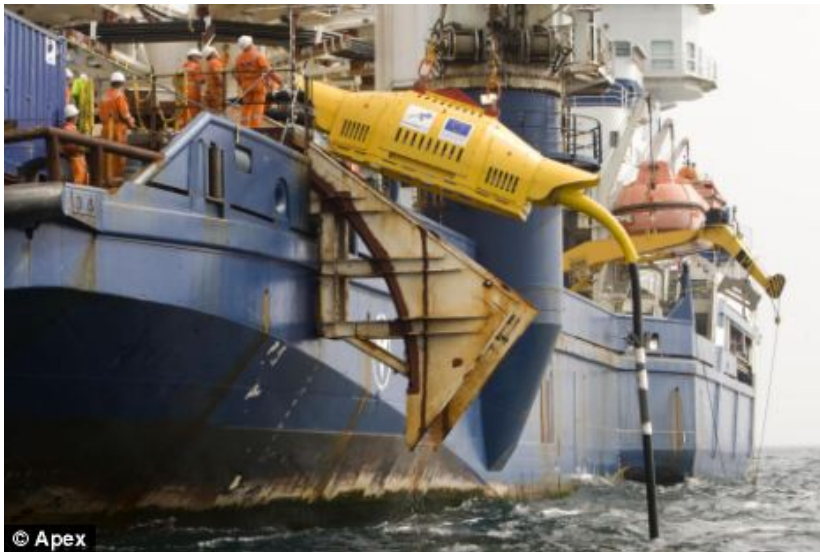
Figure 7.6 Pieces of Wave Hub are installed on the seabed following a delicate operation to lower the hub into 55 meters of water, 10 miles off Hayle, in Cornwall.
