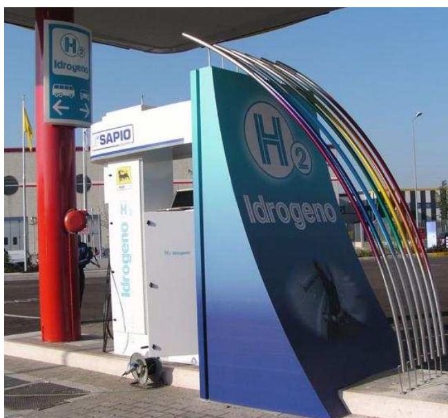
Figure 4.6 Zero Regio hydrogen refuelling unit in Mantova showing the ‘masked’ concrete wall Source: http://www.admin.zeroregio.de/CDROM/englisch/10openingeni/opening/index.html .
