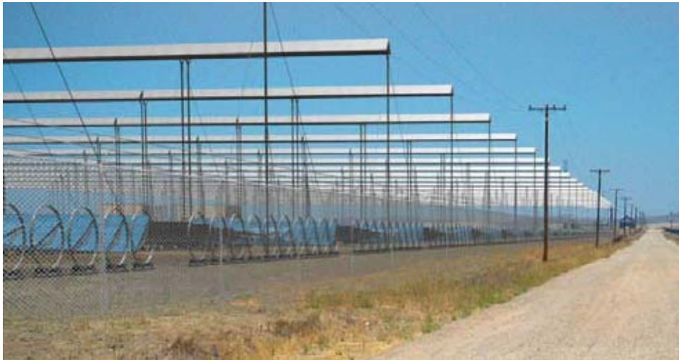
Figure 5.4 Visualisation of 177 MW e plant based on Fresnel-lens at the Carrizo Plain, CA Source: Internet Sources 28-30.
