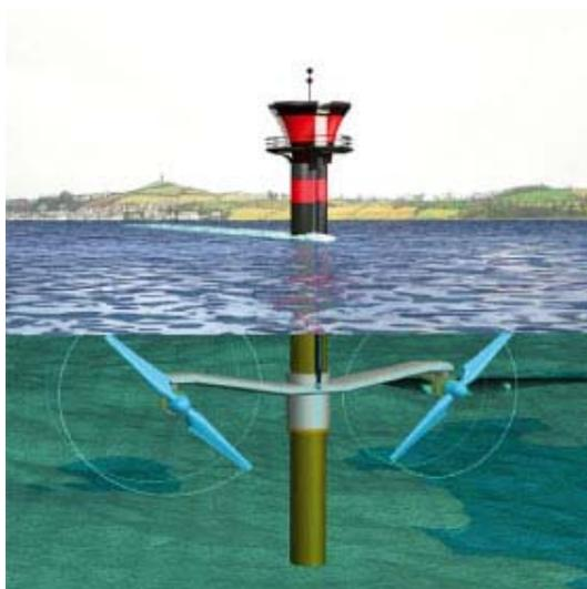
Figure 3.20 SeaGen tidal power (artist impression), Marine Current Turbines Ltd
