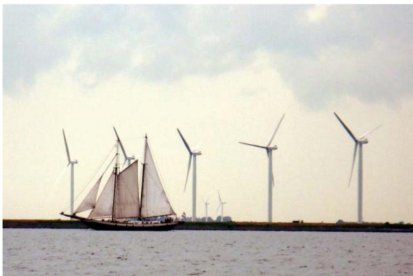
Fig. 4.1 *The EWTW test farm seen from the IJsselmeer. The turbines have a rotor diameter and a hub height of 80m and a capacity of 2.5MW each. The turbines are numbered from 5 to 9 from left to right.*
