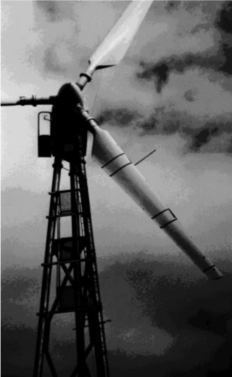
Figure 4.25 The 100 kW stall regulated wind turbine used for the RISØ experiments
