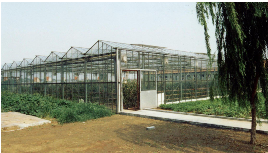
Figure 3.3 The Dutch Venlo Type greenhouse, Greenhouse III at SAHDP
