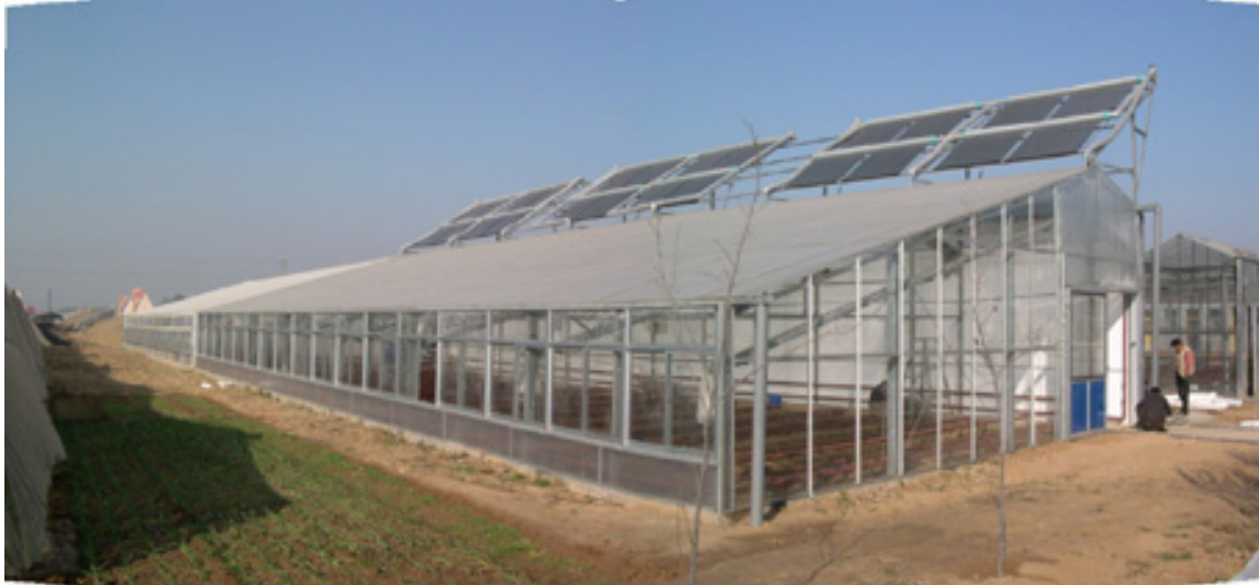
Figure 3.2 Greenhouse II (November 2004), the far left part is covered by PC board, right is covered by glass and equipped with the solar collectors
