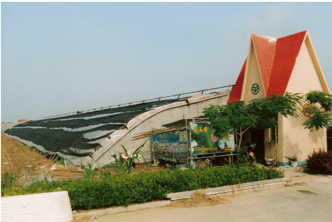
Figure 3.7 The traditional greenhouse (Greenhouse I) used for the experiments
