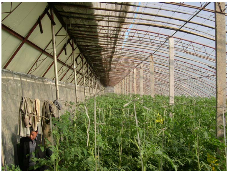
Figure 3.8 Interior of a Traditional Sunny Greenhouse
