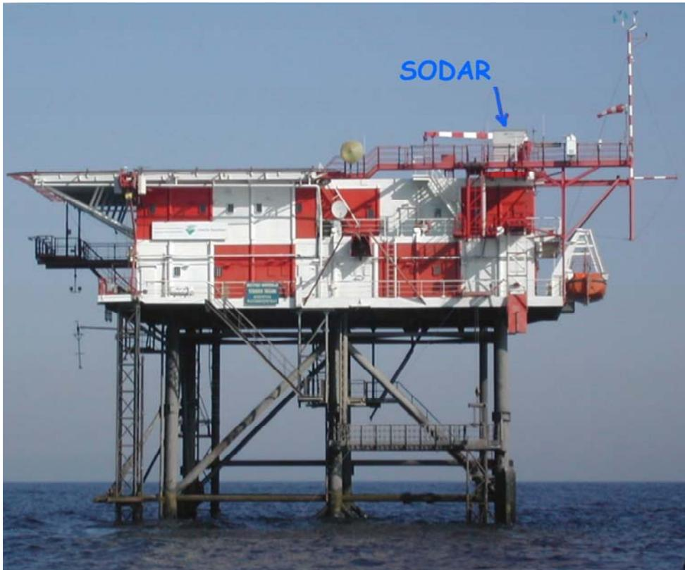
Figure 6.9. Meetpost Noordwijk (MPN), 8 km out of the Dutch shore, at the top right side of the platform the meteorological mast is located.
