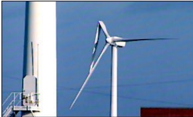
Fig. 1.1: Blade failure of an offshore wind turbine in Blyth Harbour (UK) due to a lightning strike [8,9]
